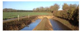
A solution: Through working together, Norfolk Rivers Trust, WWF, Coca-Cola and the Broadland Catchment Partnership funded the construction of three large roadside sediment traps to slow the flow of water, allowing soil and sediment to settle in the traps and reducing the amount reaching the river.
